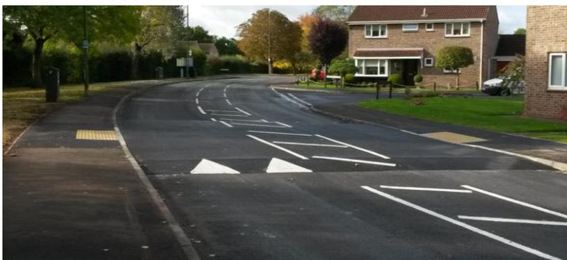
Speed tables are a raised section of road, with a ramp on both sides. The ramps are painted with white arrows to make them more obvious to motor vehicle drivers.
