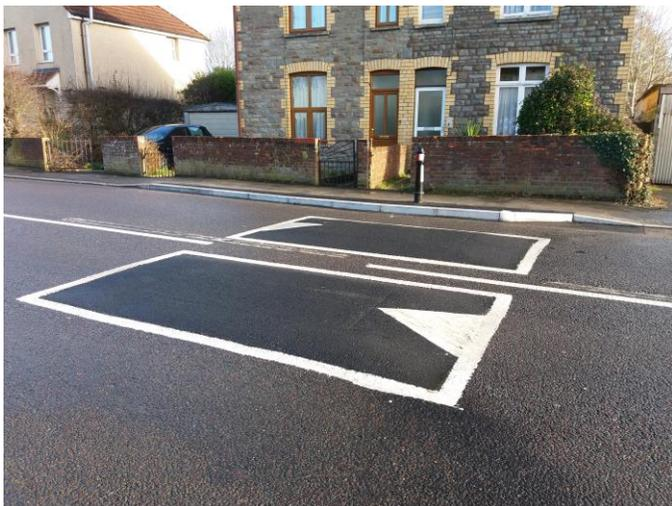
A speed cushion is a short, raised, rounded device, normally in the centre of a road lane. Speed cushions are designed to be slightly wider than a car, so car drivers need to slow down and drive over the centre of the speed cushion to minimise the effect. Buses are wider than cars, so they can drive over speed cushions without passengers feeling it.
