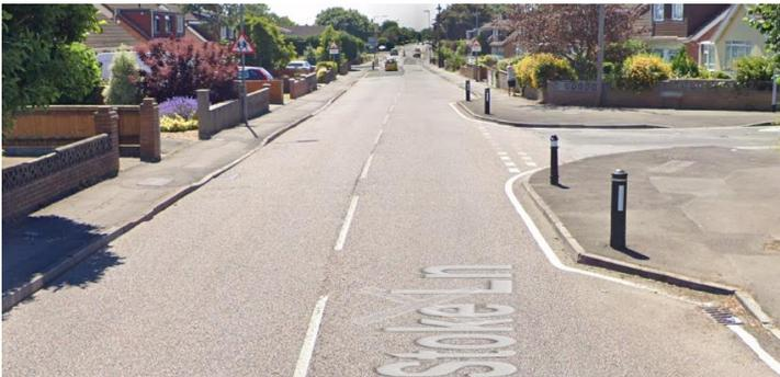
A road narrowing simply reduces the width of the road on one or both sides.
